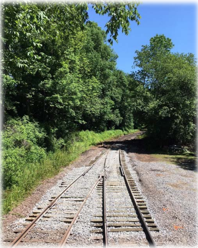
Halcottsville Switch Project nearing Completion
